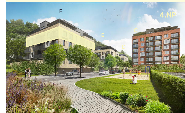
Pohled na dům / Building View
