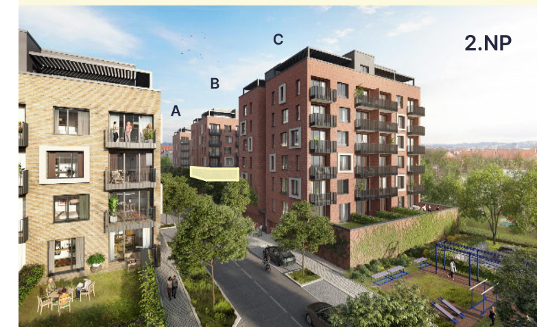
Pohled na dům / Building View
