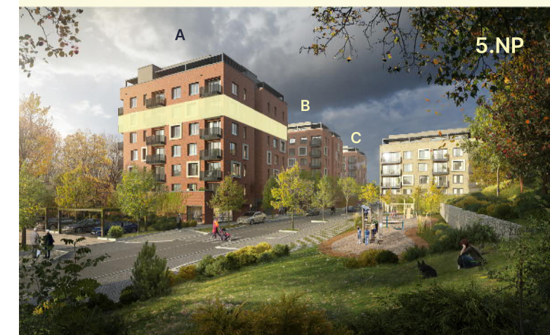
Pohled na dům / Building View
