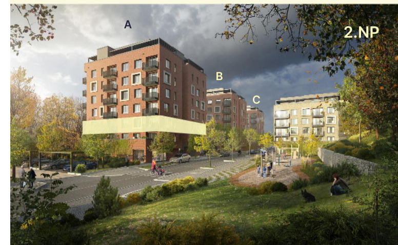
Pohled na dům / Building View
